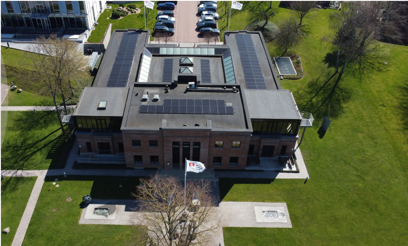
Bunker Holding headquarters in Middelfart, Denmark, powered by solar panels installed in 2022
